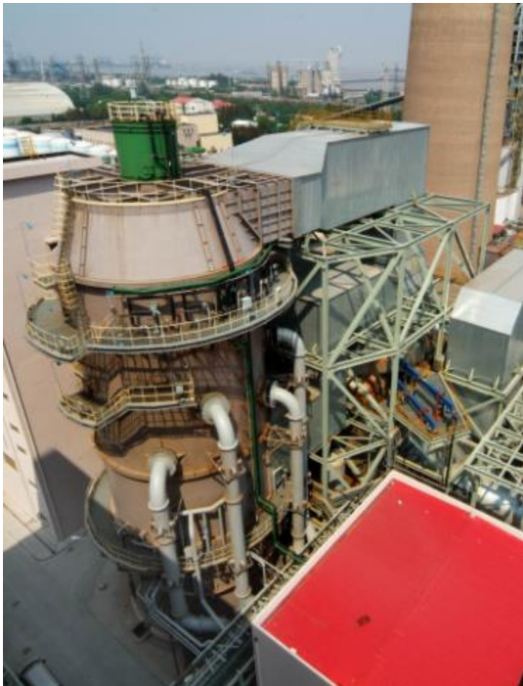
Baogang Power Plant 3x350MW Retrofitting project Time of Commission: 2008-2009
