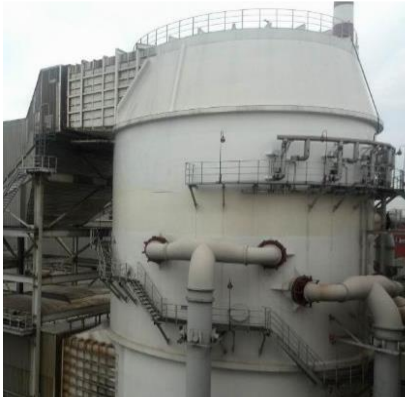
Waigaoqiao 2 Power Plant 2 × 900MW Retrofitting project
